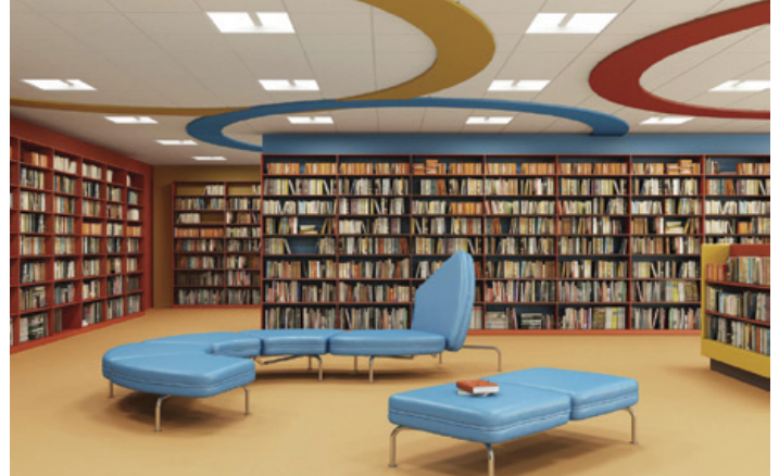
Eaton LED light fixtures and UPS solutions work together in libraries and other public spaces to keep patrons safe.
