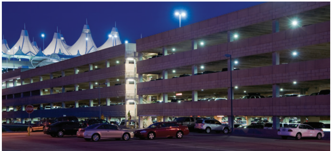
At the Denver Airport, Eaton lighting equipment ensures the parking facilities are illuminated and safe at all times.
