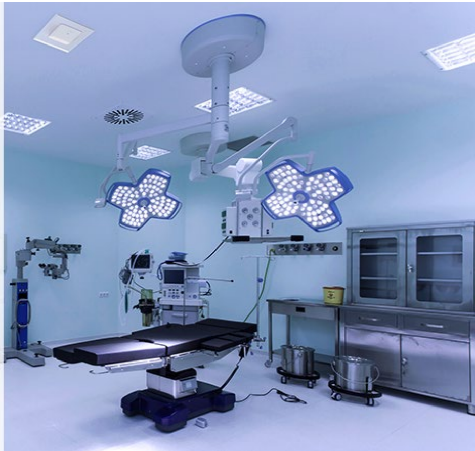
These types of openings in the ceiling tile are undesirable in a healthcare environment.
